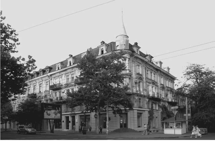
FIGURE 1. The Babel family apartment in Odessa (the top floor above the billboard) at the corner of Rishelievskaya and Zhukovskogo, where Babel resided in 1906–1911 and, on and off, in 1919–1924. Photo © by Gregory Freidin.
